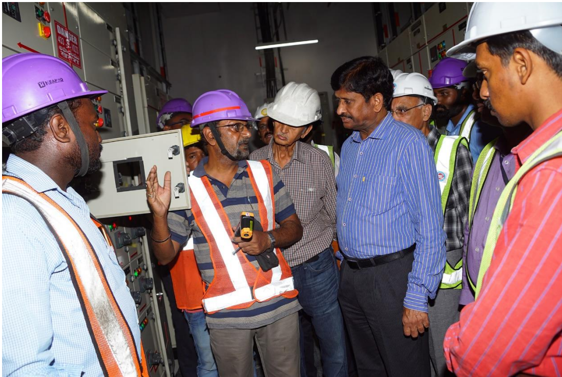
Image 2 - Mr. DVS Raju, CEIG along with other officials inspecting the Auxiliary Substation
