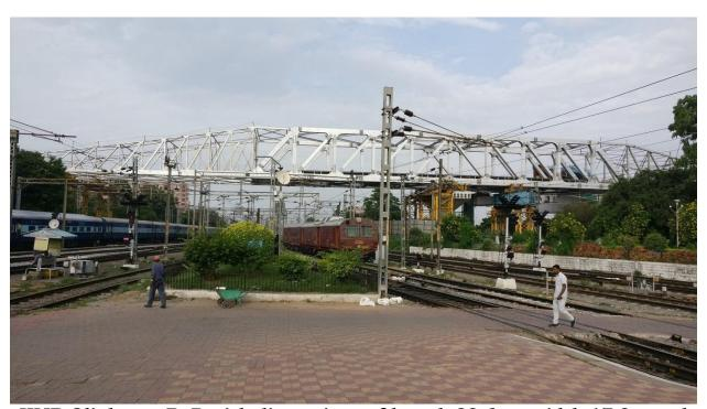
HMR Oliphenta RoB with dimensions of length 82.6 m, width 17.3m and height 10.55m spanning across 8 existing and 5 future tracks.
